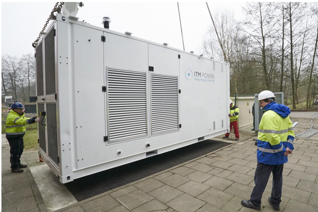
ITM Power-to-Gas PEM electrolyser system
