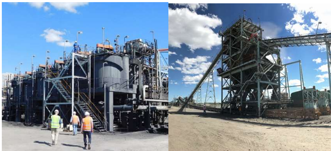
Flotation and crushing plants at the Mowana Copper Mine. Source: Company
