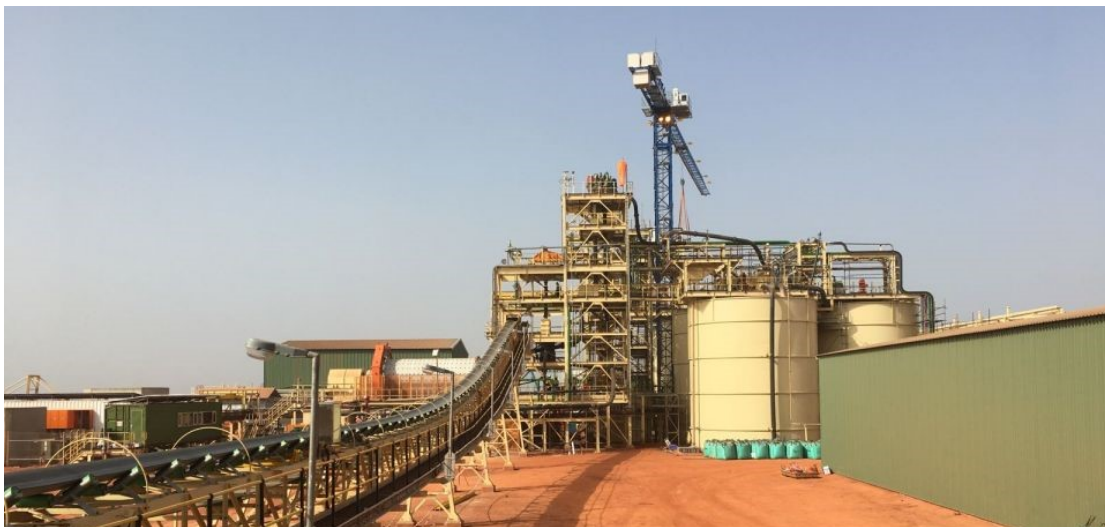
Mill during construction. Source: Company
