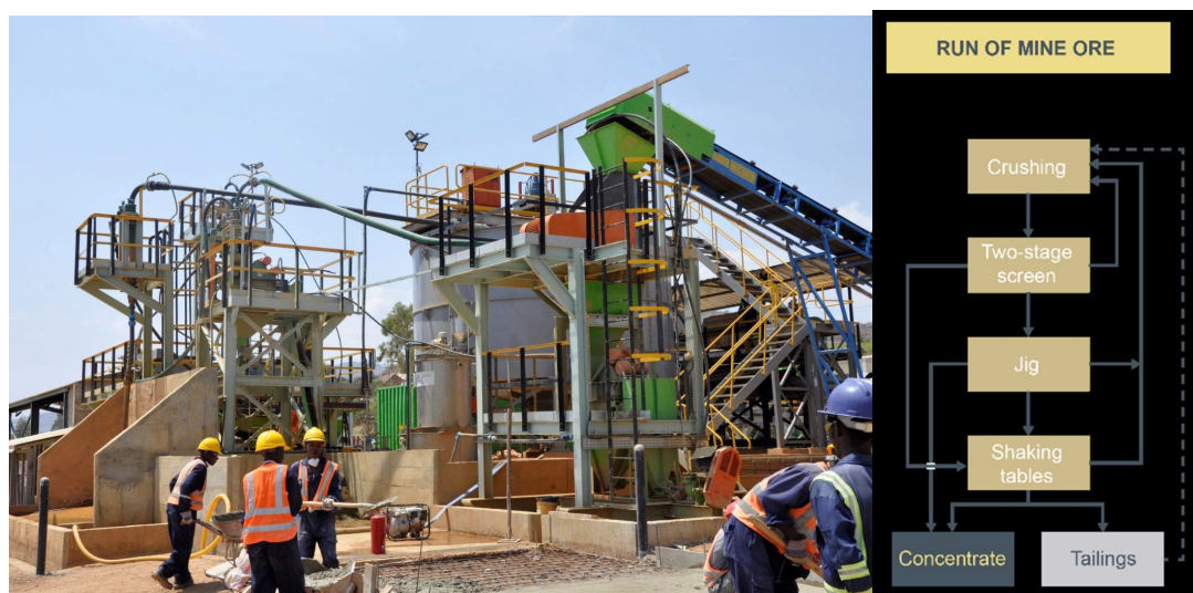
Kabezi processing plant and the flow chart for the mineral processing. Source: Company
