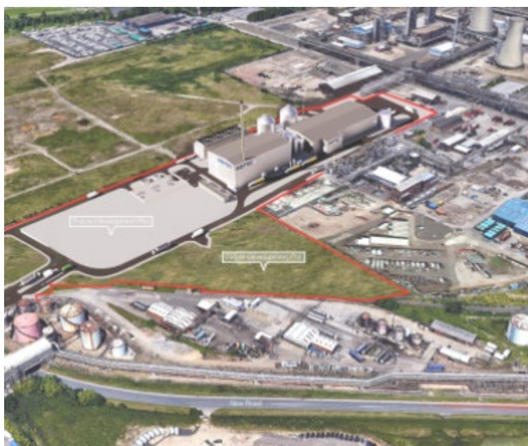
Billingham site. Source: Company
